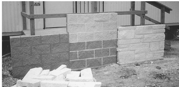
Figure 17-4 Traditional masonry sample panels for evaluating unit color, color range, mortar color, joint tooling, and general workmanship.
